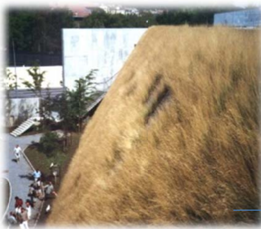
Wall, first spring after planting
