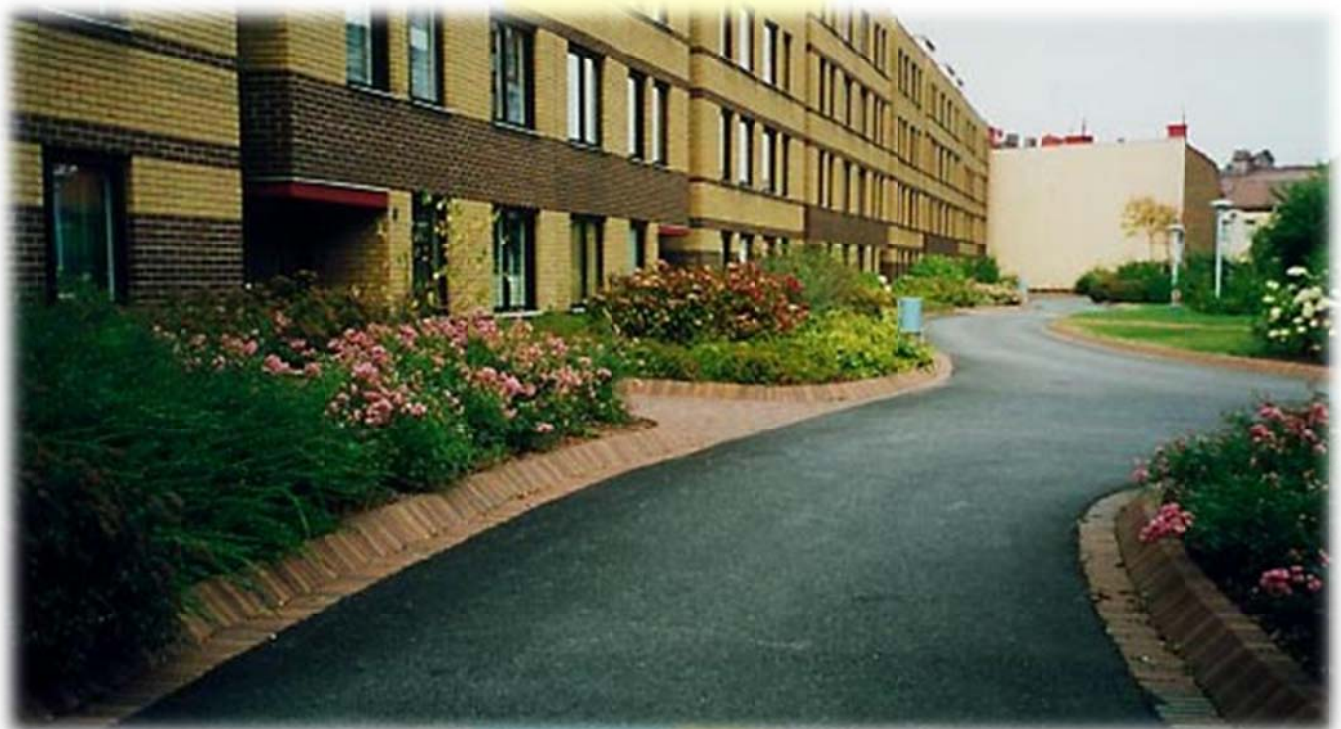
Fig. 3 Nilssonsberg project, Goteborg, Sweden
